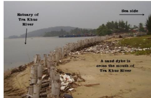
Fig. 3. Staking to prevent the accumulation of sand from the sea into the Tra Khuc River (Quang Ngai).
