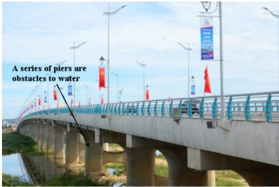
**Fig. 13.** A series of piers are obstacles to water, reducing the ability to drain water on Tra Khuc river.
